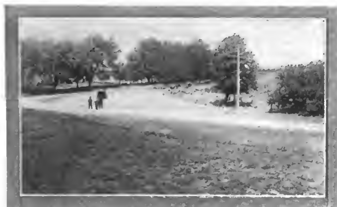
The turn at Udina, formerly the worst on the course, has been widened to 80 feet
